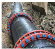
The Tite Liner® system is suitable to connect to all types of piping systems (DIP, CS, PCCP, AC, HDD, etc). Fittings, valves and miters can be accommodated with HDPE, DI, CI or other materials and bolt directly to the Tite Liner® system.
