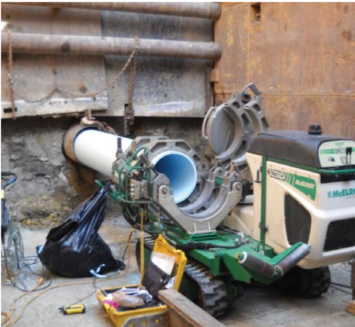
Slipline/Jack and Bore
