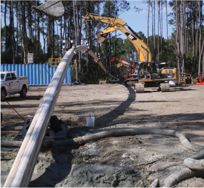
Horizontal Directional Drill
