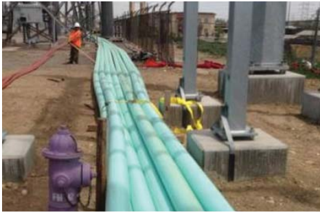
Cherokee Power Station Denver, CO
