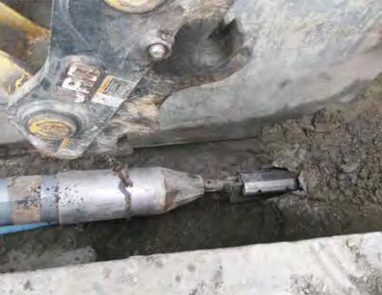
*Cutter Tooling and Expander Head Entering Host AC Pipe*
