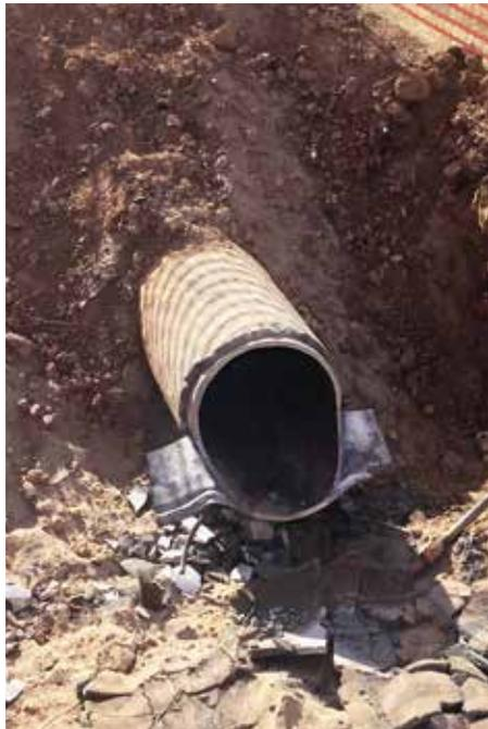
Existing 18-inch concrete lined steel water pipe had an I.D. of 17.5 inches
