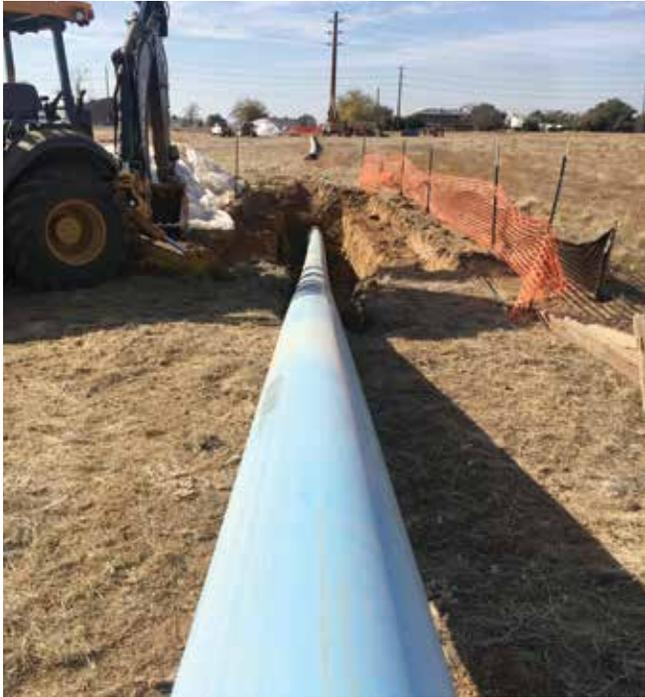
Pipe was installed in typical run lengths of 500-1,000 feet
