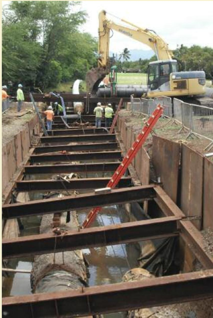
*Pulling the new 24" Fusible C905 pipe into the borehole while working over existing meter station and Caltrans signalized intersection.*
