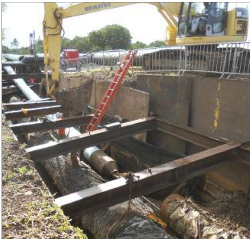
*Pulling Fusible C905 over the adjacent drainage channel and into the 30-inch force main*
