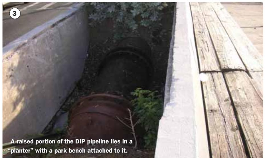
A raised portion of the DIP pipeline lies in a "planter" with a park bench attached to it.
