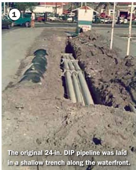
1 The original 24-in. DIP pipeline was laid in a shallow trench along the waterfront.
