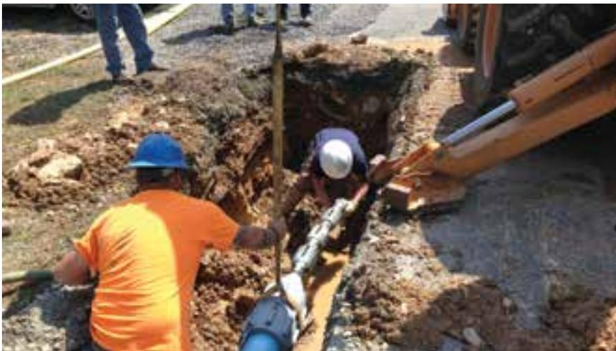
Photo 5: In Roanoke Rapids, 6" DR18 Fusible PVC® pipe entering pit for pullback.
