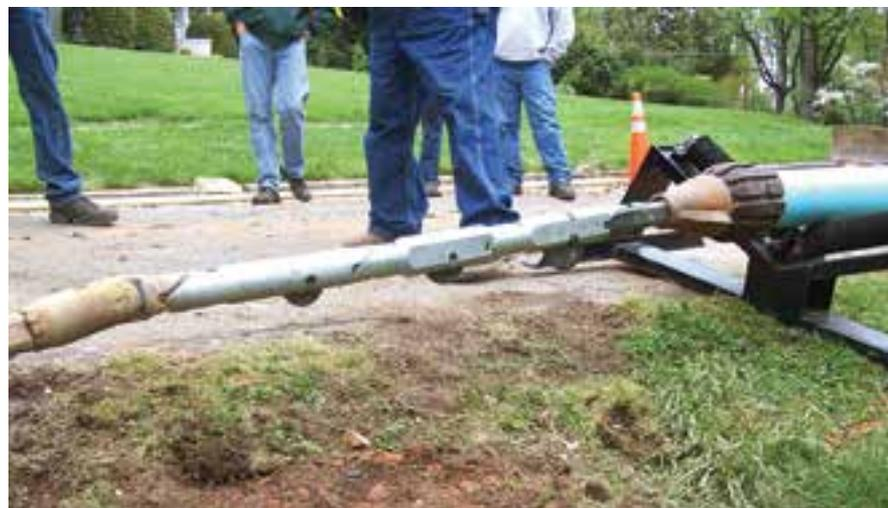
Photo 2: In Wilmington – Back end of TT Technologies 1900G with rod removal during pullback.
