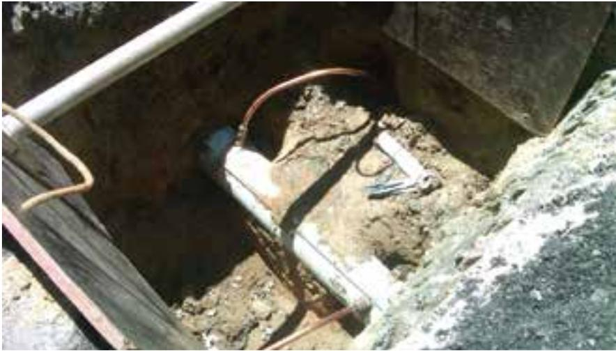
Photo 4: In Monroe – Pipe attached to expander head, in turn attached to cutting wheel tooling.
