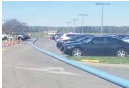
*Fusible PVC® pipe is staged through a parking lot for just a few hours before installation begins*
