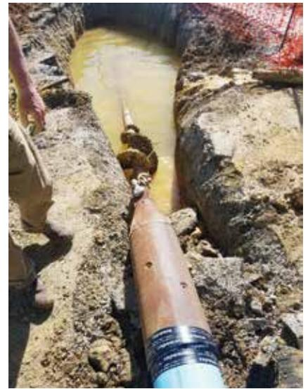
*Final reaming and insertion of the Fusible PVC® pipe occurred simultaneously*
