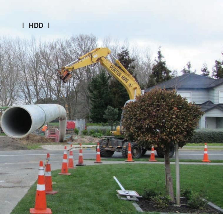
Successful water filled pipe string ballasting techniques were utilised on the New Zealand case study.
