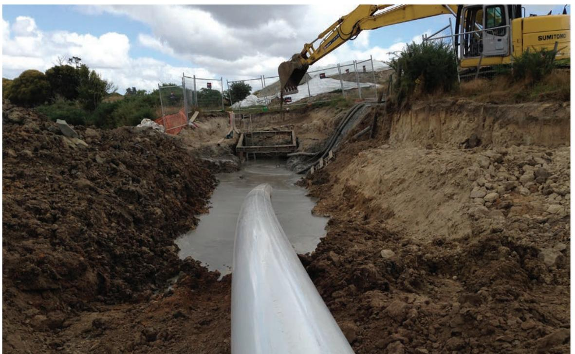
**Opposite page:** Installation of DN475 SN16 FPVC being pulled in an urban environment.
