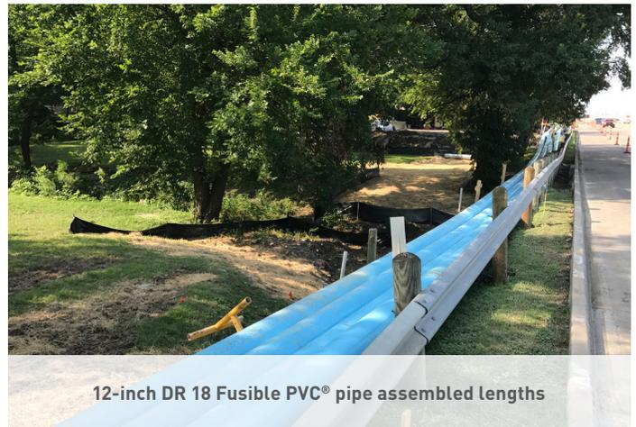
12-inch DR 18 Fusible PVC® pipe assembled lengths
