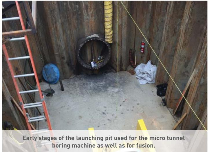
Early stages of the launching pit used for the micro tunnel boring machine as well as for fusion.
