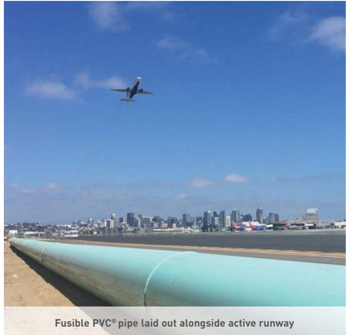
Fusible PVC® pipe laid out alongside active runway
