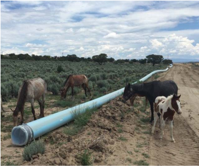
Navajo Nation 14" DR18 Fusible PVC® water main ready for installation
