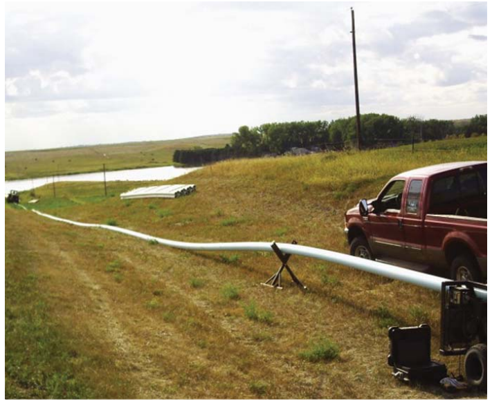
Spirit Lake Nation 8" DR14 Fusible PVC® water main
