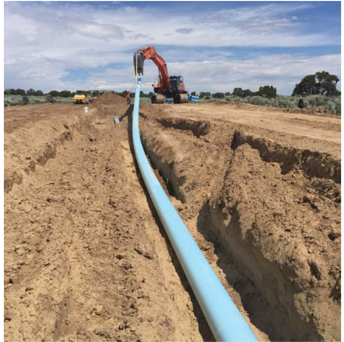
Fusible PVC® pipe in The Navajo Nation
