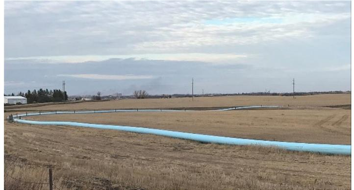
Fusible PVC® pipe ready for installation of a 3,000-foot HDD
