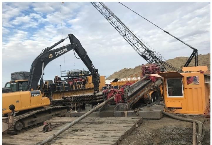
Horizontal directional drilling rig layout
