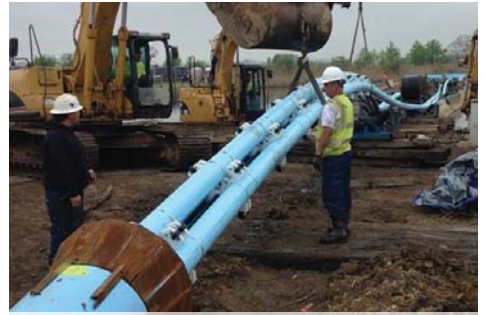
Woodbridge, NJ: 11,000 LF of 30" Casing
