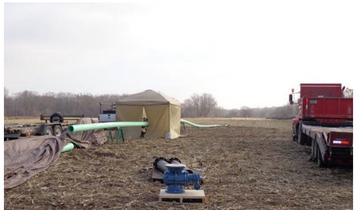
Layout and cold weather (December) fusion
