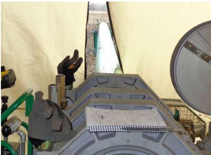
Each joint is data logged and recorded
