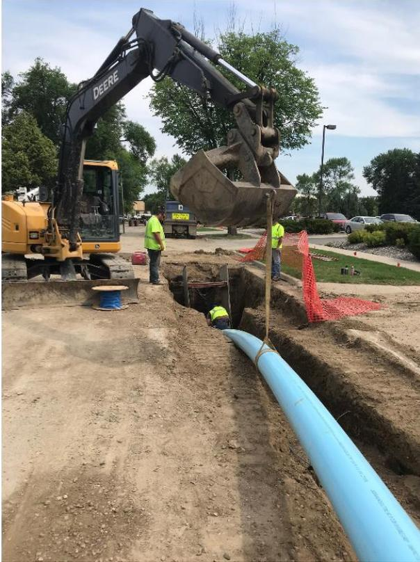
Figure 7: Fusible Pipe laydown in for 6<sup>th</sup> St S Water main Replacement Project
