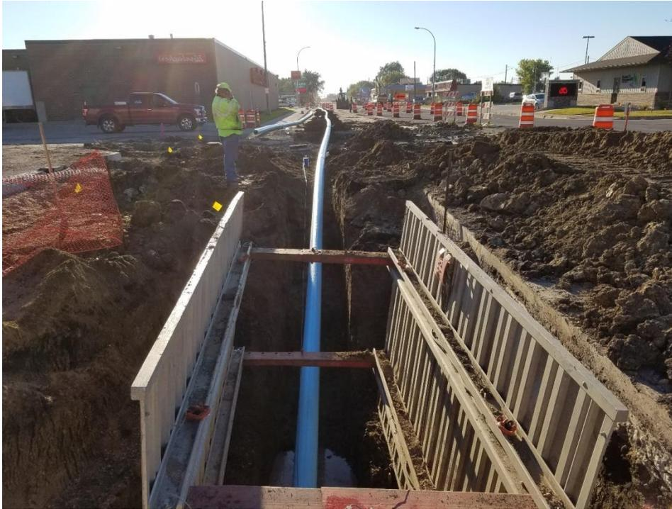
Figure 3: Fusible Pipe laydown in CIMS Project
