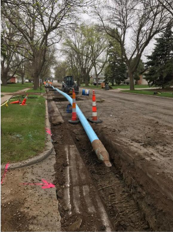
Figure 4: Fusible Pipe laydown in Southside Project
