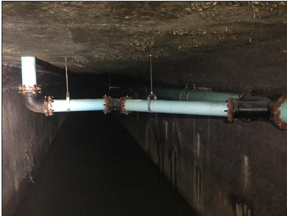
Figure 9. Existing trunk sewer with new force main pipe mounted on brackets and a wye to a 6-inch service lead for potential Coca-Cola connection.
