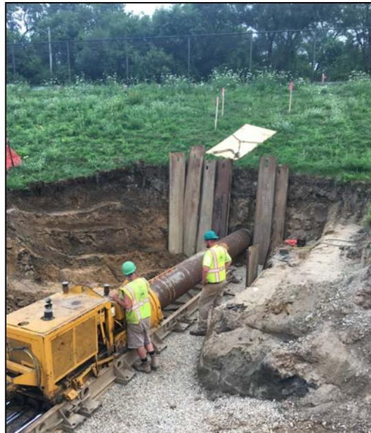
Figure 4. Jack-and-bore installation of pipeline
