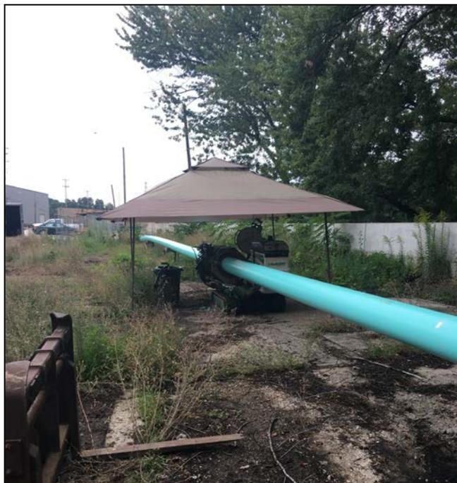
Figure 6. Canopy set up to shield fusion process from rainy weather and pipe fusion continued as normal.
