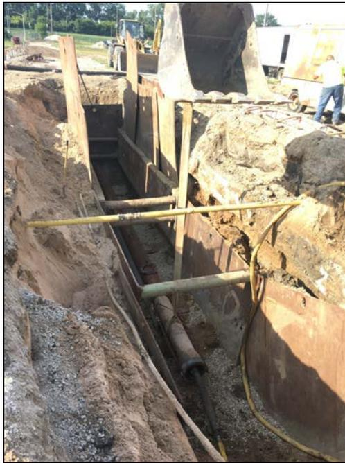
Figure 5. Pipe ramming near the connection to the WRRF.
