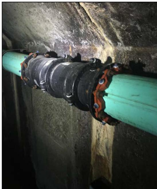
Figure 8. Expansion joint installed along wall-mounted force main in trunk sewer.
