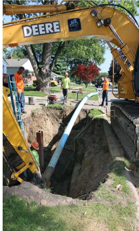
Figure 5. Pulling Operation; Tension Line and New Pipe
