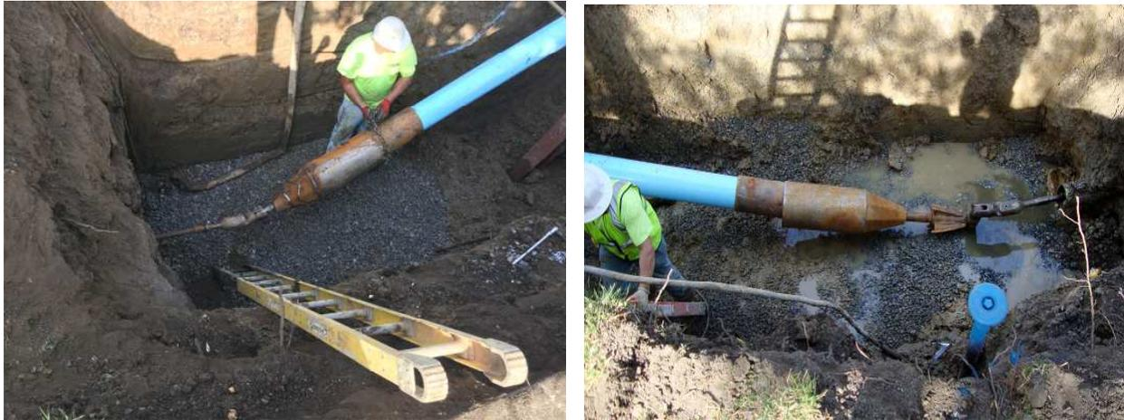
Figure 4. Pipe Bursting Head
