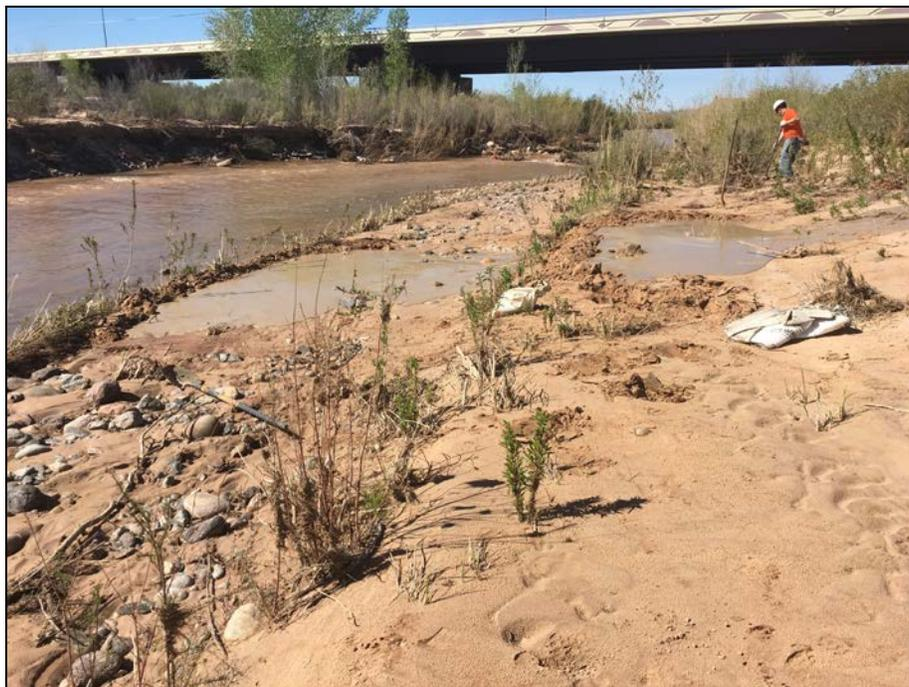
Figure 6. Release of bentonite as a result of minor frac out event.
