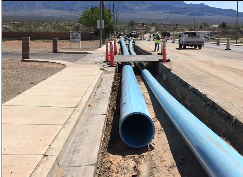
Figure 7. Carrier and casing pipe fused and ready to pull in.
