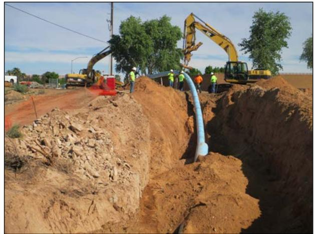
Figure 10. Carrier pipe being pulled into the casing pipe. Initial insertion (left) and alignment around the tree to the insertion point (right).
