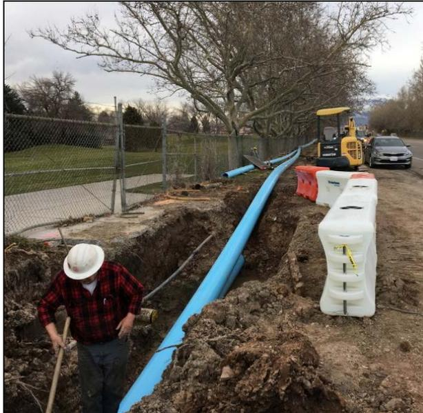
Figure 9. Pipe insertion pit between 12-inch pipe burst runs.
