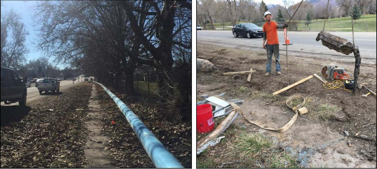
Figure 7. Setup along Washington Blvd bursting hardware being placed into position (right).
