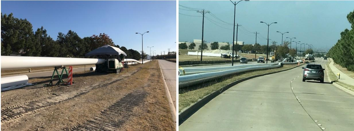
Figure 5. The median provided ample layout space [FPVCP fusion and staging (left); FPVCP layout (right)].
