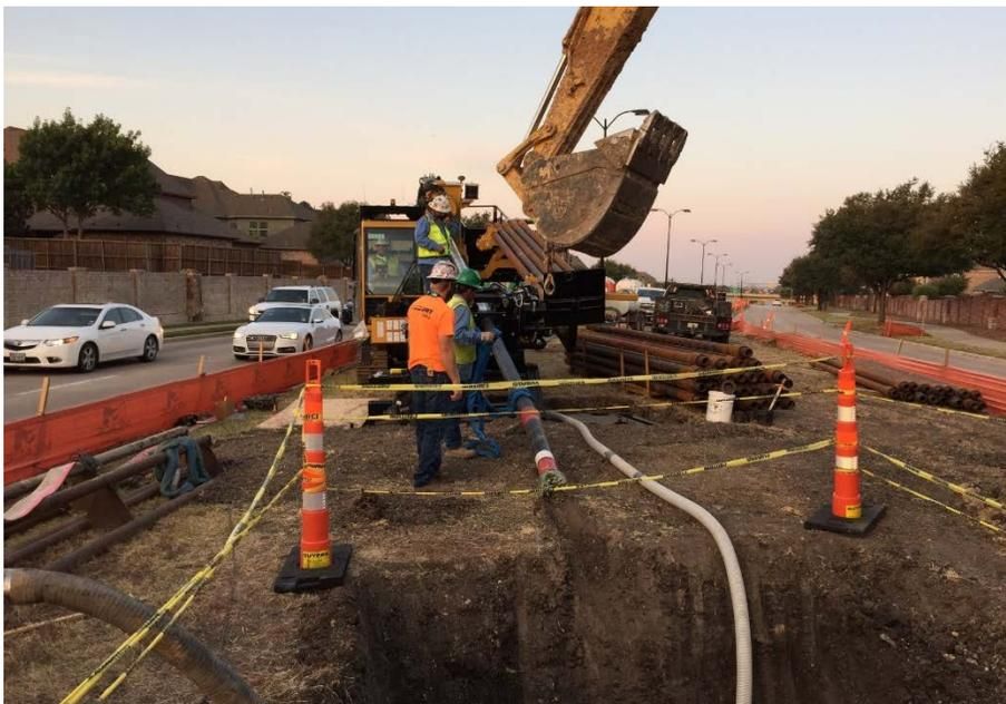
Figure 6. Vermeer 220x300 drill rig being set up to drill the pilot hole.
