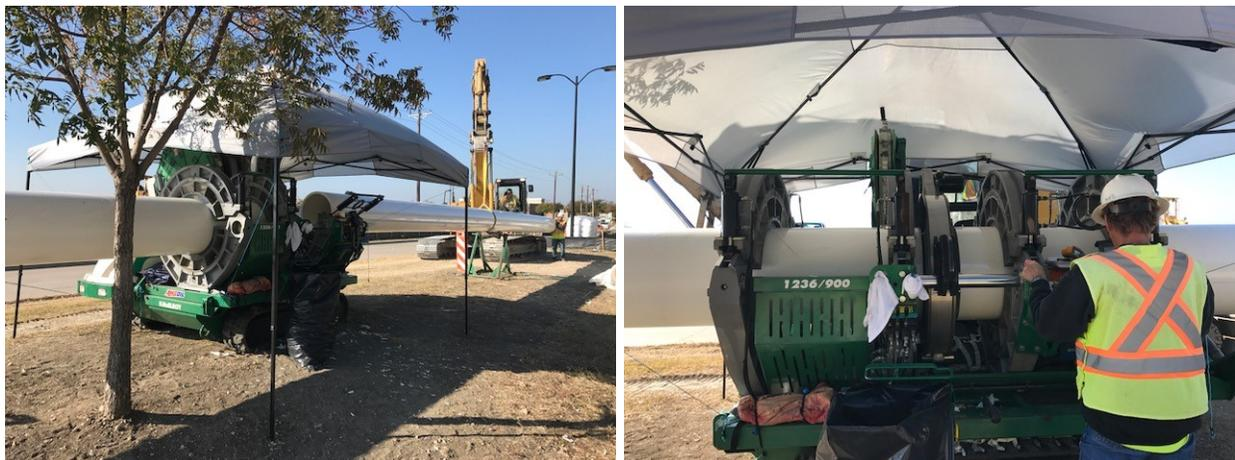
Figure 4. FPVCP fusion, individual FPVCP stick being inserted into fusion machine (left); certified fusion technician fusing FPVCP into one continuous length (right).
