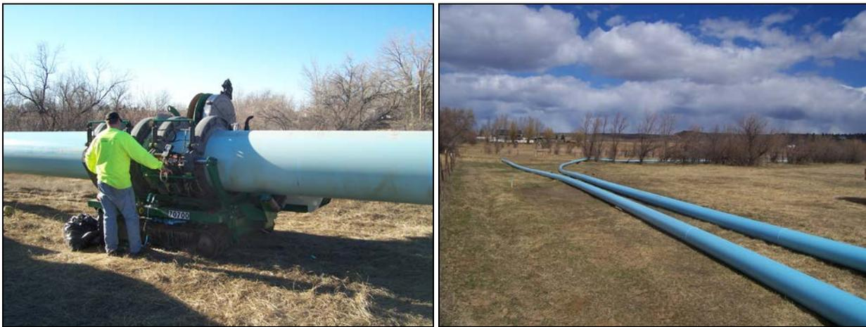
Figure 5. Project location had ample open area for staging and pipe layout [fusion (left); layout (right)].
