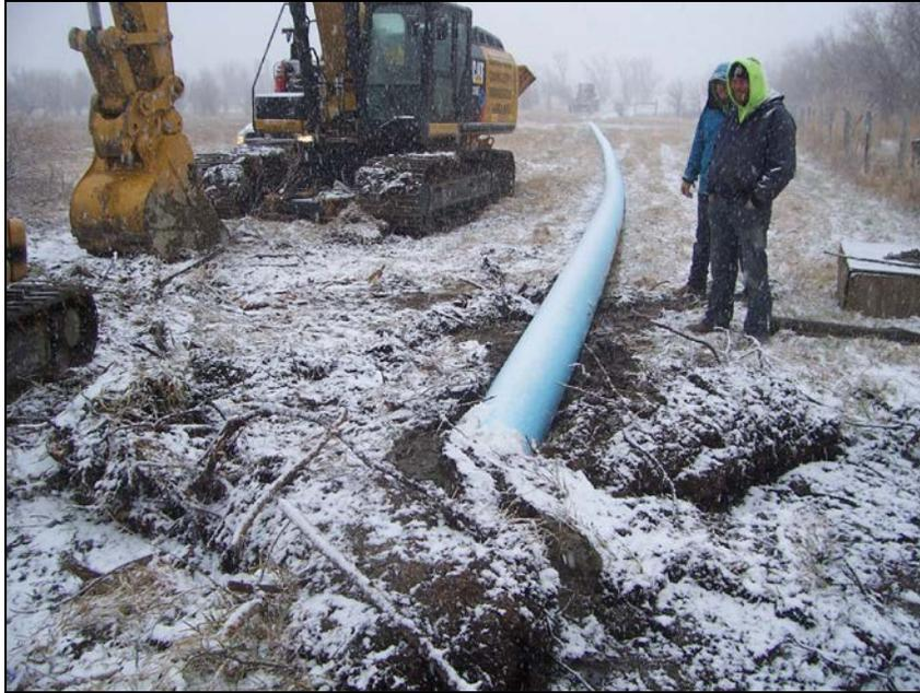
Figure 6. HDD pull-in under tree grove. The bore was installed in cold and inclement weather.
