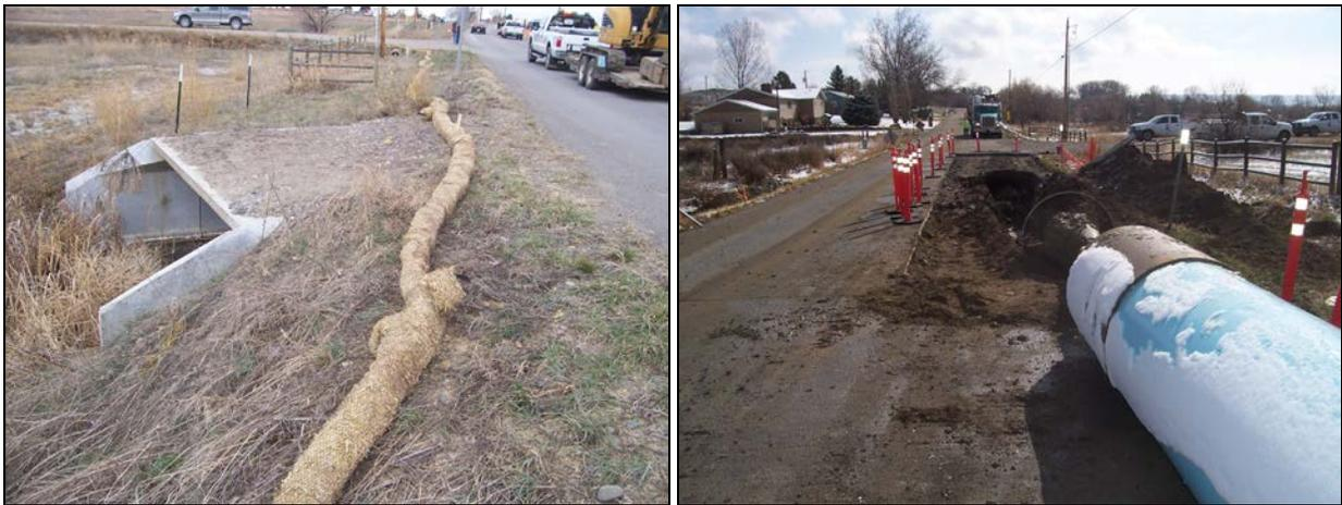
Figure 7. Staging and installation of crossing under box culvert [existing culvert (left); pull-in (right)].
