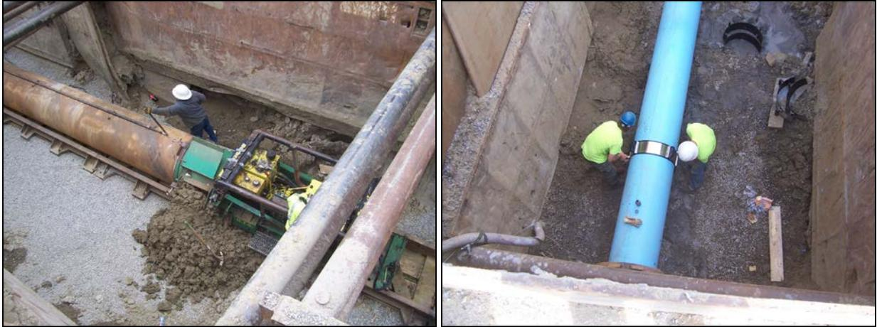
Figure 8. Jack-and-bore installation under Phillips 66 oil pipeline. A steel casing was bored and jacked into place (left); FPVCP with casing spacers was then placed inside the casing (right).
