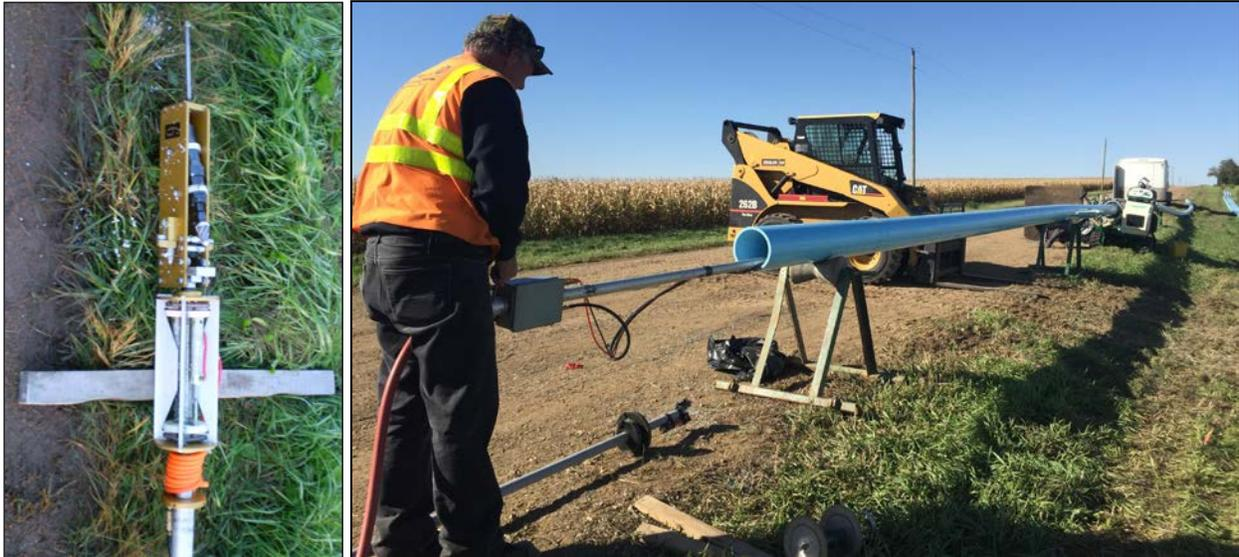
Figure 6. Internal debanding of FPVCP casing [internal debanding tool (left); debanding process (right)]
