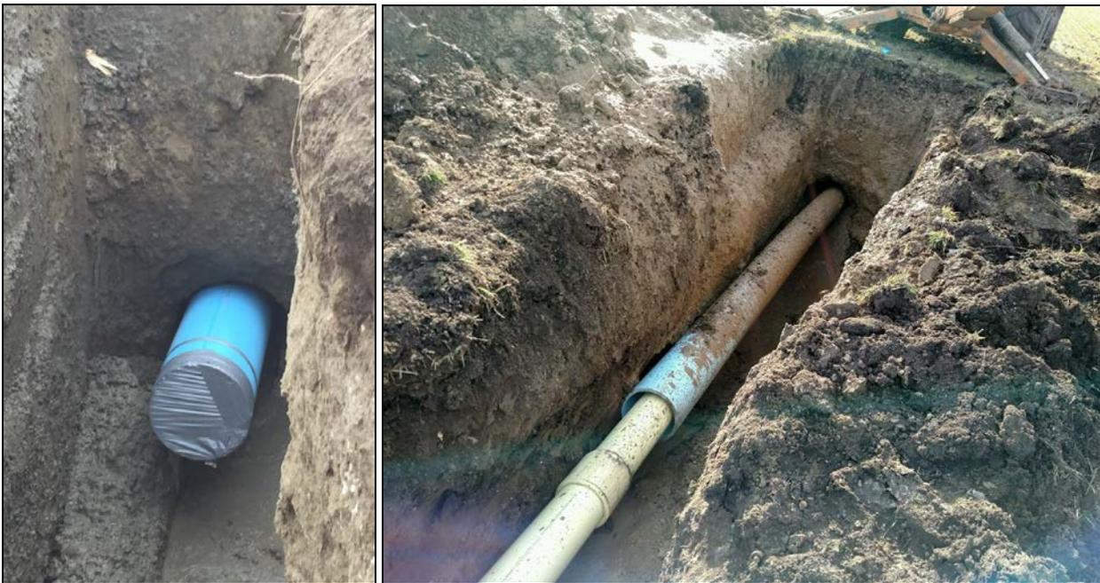
Figure 7. Casing and water line installation [installed casing pipe (left); insertion of carrier into casing (right)]
