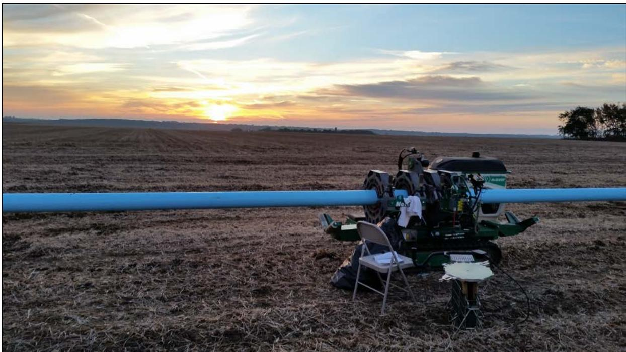
Figure 3. Casing pipe fusion in South Lincoln Rural Water System.
