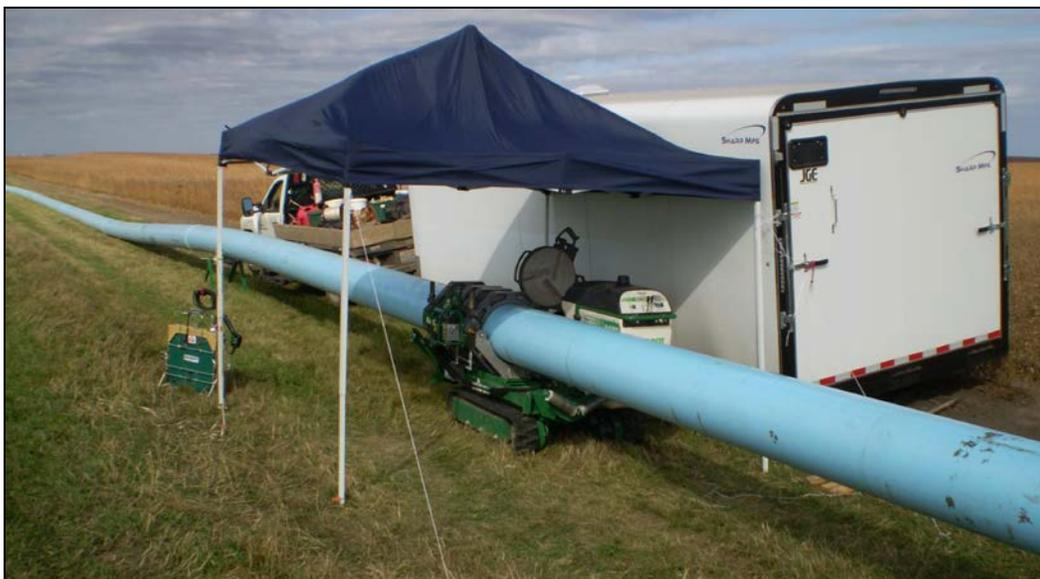
Figure 5. Fusion setup by Dakota Directional in Web Water Development.
