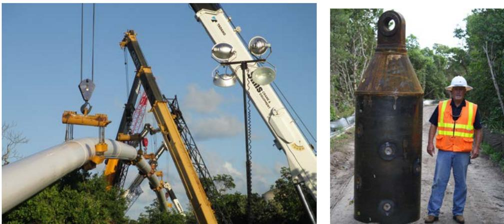
Figure 5. (left) Cranes were used to cradle, align, and direct the pipe above the mangrove area. (right) Pull head used to install both casings.
