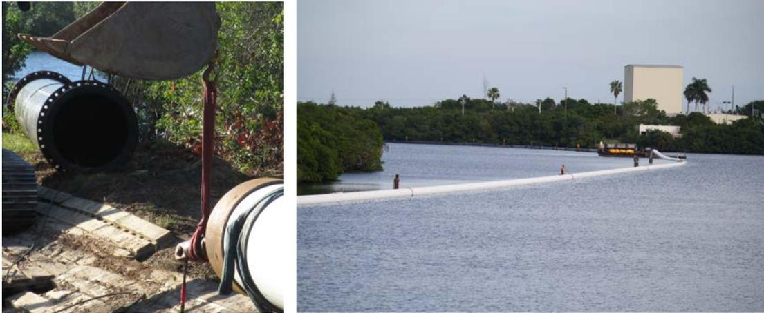
Figure 4. (left) FPVCP casing prepares to enter HDPE culvert. (right) FPVCP pipe exits culvert, floated across creek.
