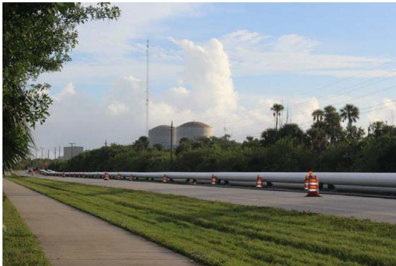
Figure 3. Assembled casing layout on rollers along the west shoulder of A1A.
