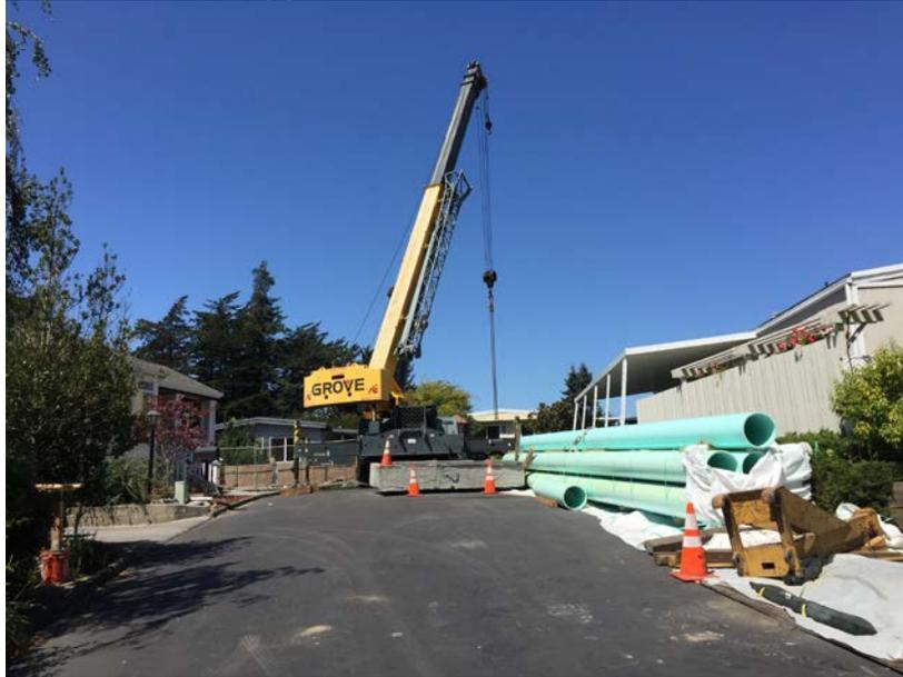
Figure 9. Installation of carrier pipe in tight corridors
