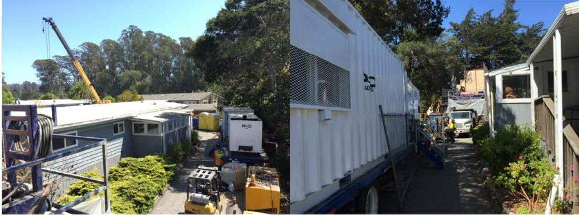
Figure 6. Micro-tunneling support equipment in tight corridors around 45' deep jacking pit
