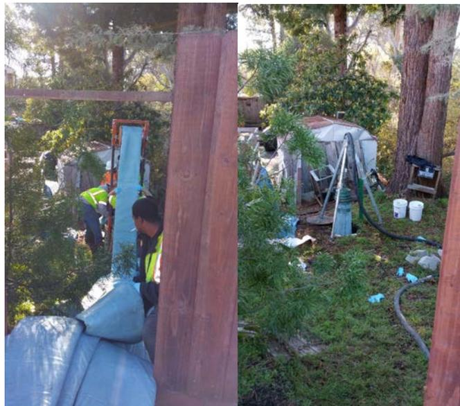
Figure 7. Installation of cured in place pipe behind residential homes within the gulch.
