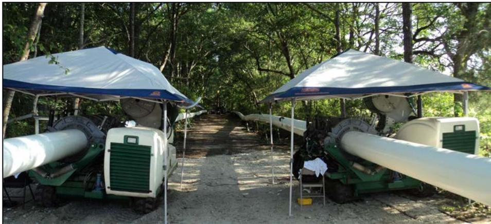
Figure 8. Fusion of 16-inch DR 14 FPVCP using two T-90 machines simultaneously.
