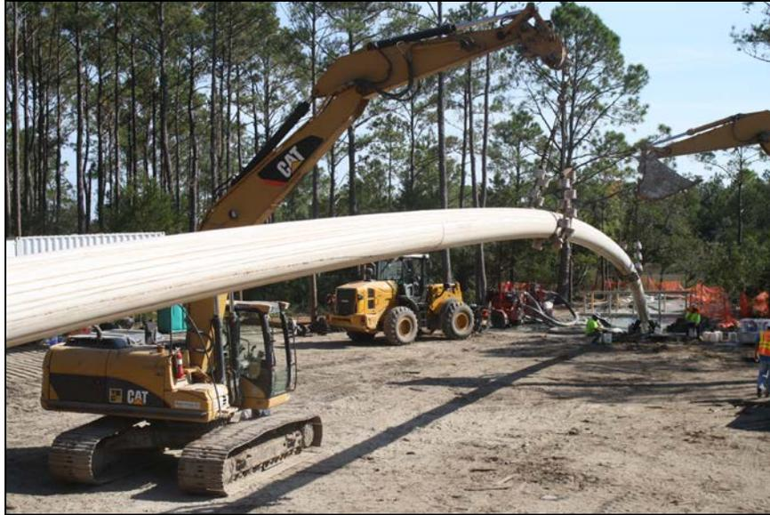
Figure 9. Aerial insertion into the bore under Kiawah River.
