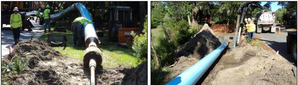
Figure 5. Pullback under lagoon on Kiawah Island [aerial insertion into HDD exit (left); pull into borehole (right)].
