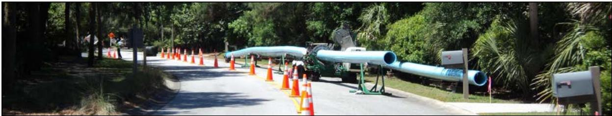
Figure 4. Traffic control for lane closure to fuse FPVCP strings.
