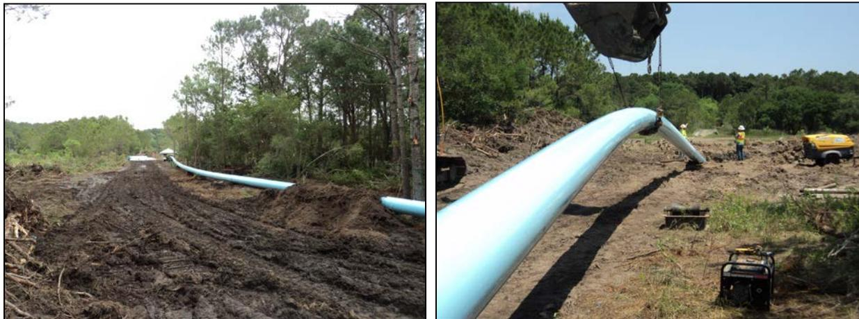
Figure 7. Layout and installation under Chaplin Creek on Johns Island [curved layout (left); aerial insertion (right)].
