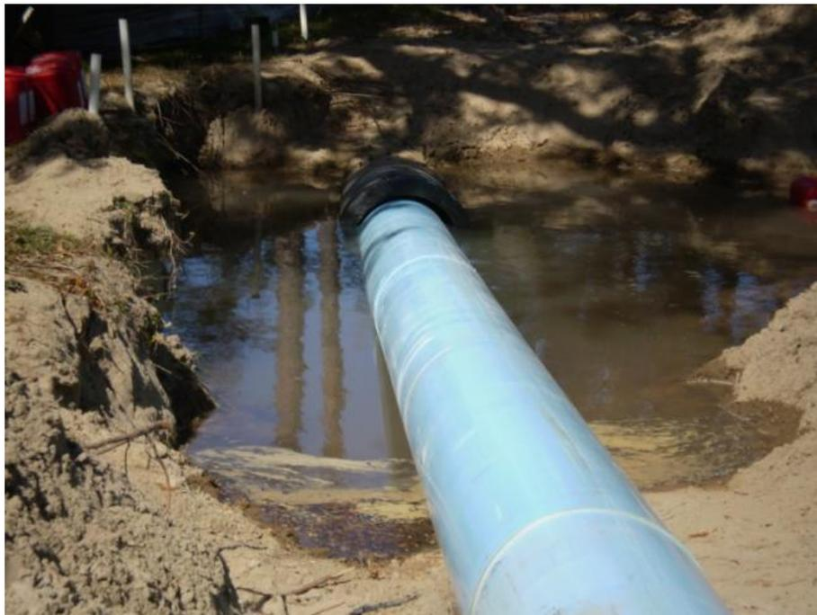
Figure 6. 20-inch FPVCP water main entering existing 30-inch DR 9 DIPS HDPE water main during slipline operation.
