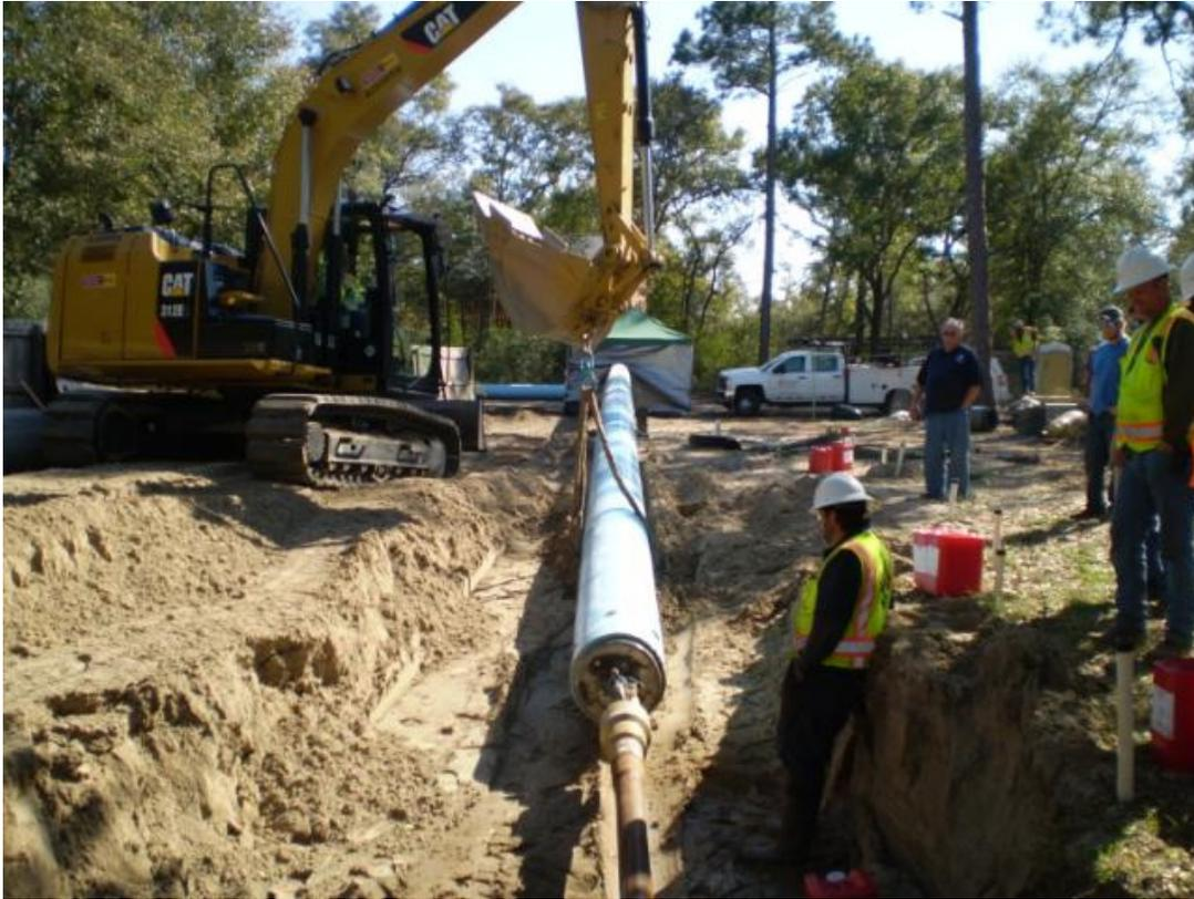
Figure 7. Fuse-and-pull operation and initial slipline insertion of Fusible PVC® Pipe
