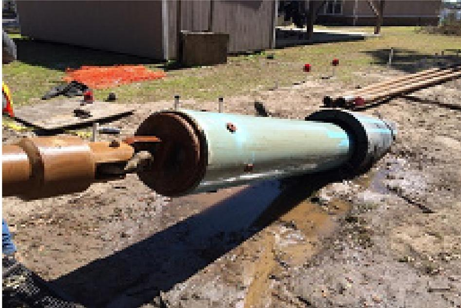
Figure 5. Internal pull-head attached to 20-inch FPVCP, shown here exiting the host pipe.
