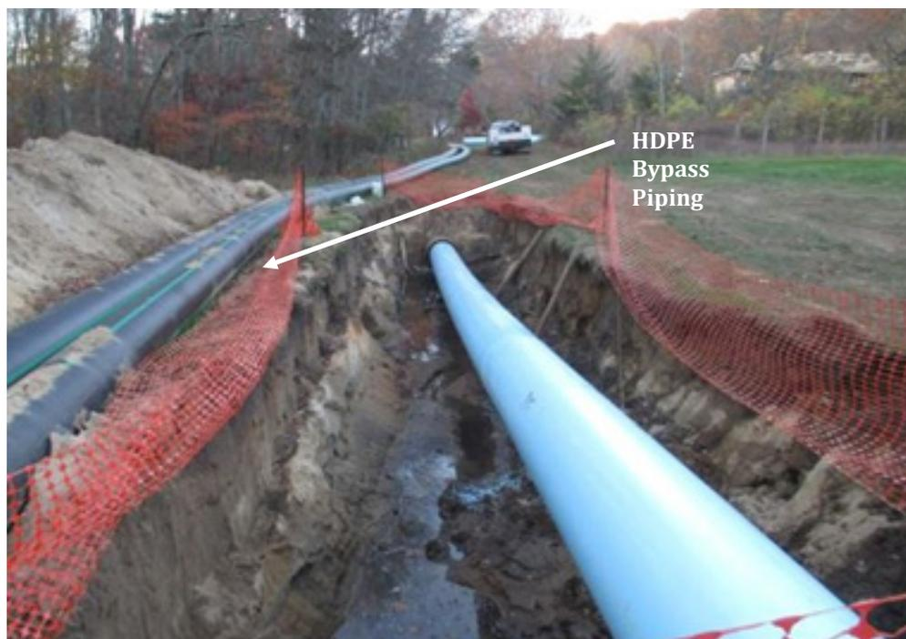
Figure 2. Installed bypass piping laying at grade along the existing transmission main alignment.
