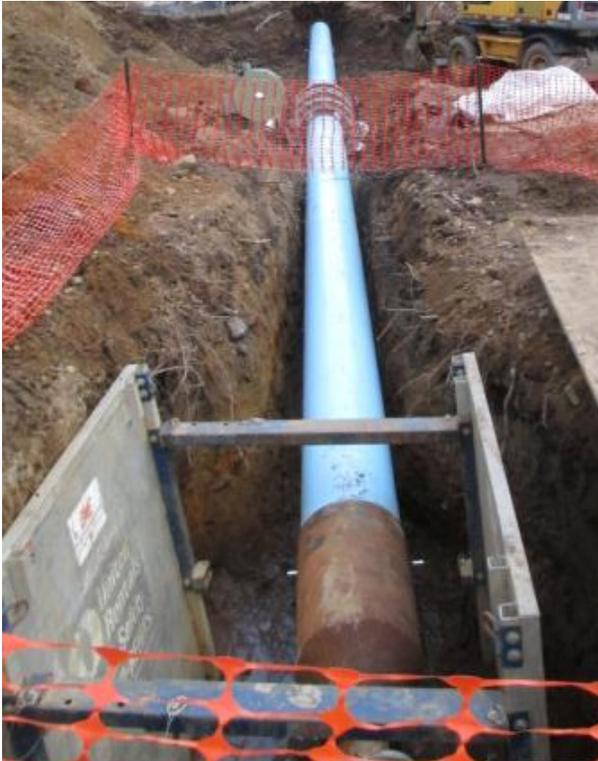
Figure 4. In-ditch fuse-and-pull installation.
