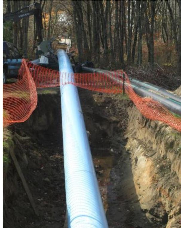
Figure 5. Aboveground fuse-and-pull installation.
