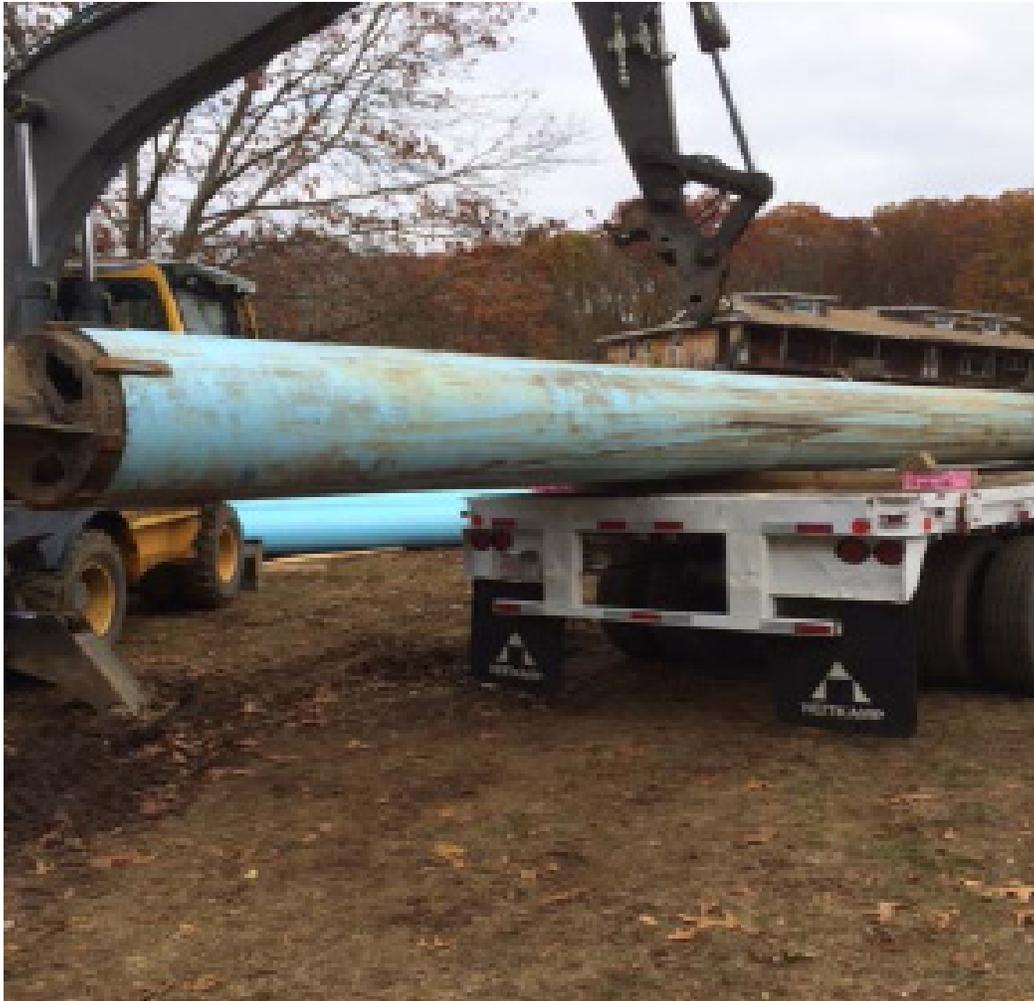
Figure 3. “Proof” piece of pipe after travelling 3,500 LF through the existing cast iron pipe.
