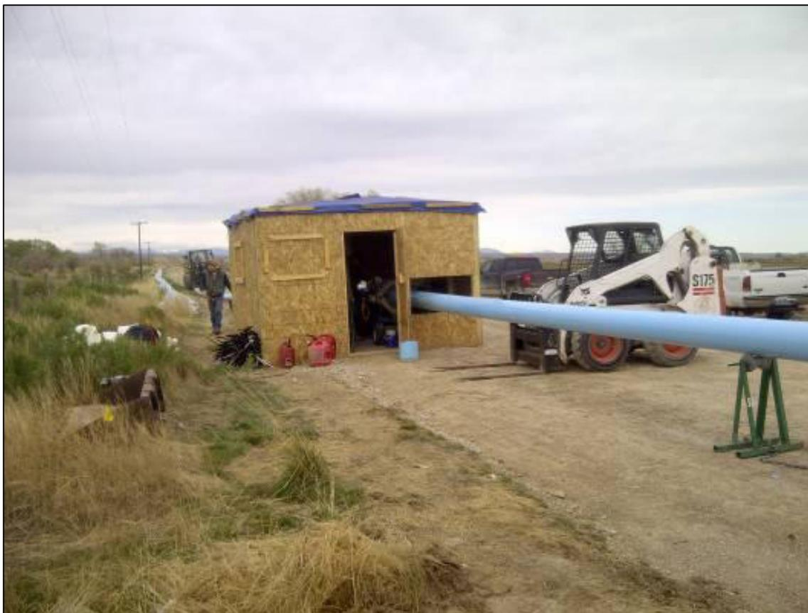
Figure 5. Fusion protection from Wyoming elements
