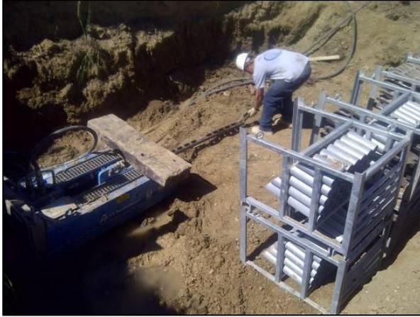
Figure 6. Insertion of pipe burst rods
