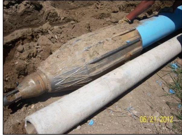
Figure 7. Pull head on 10-in Fusible PVC® pipe next to 6-inch Asbestos Cement pipe
