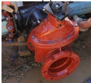
**Figure 11 - Mechanical Joint Fittings & Restrainer Glands**
