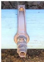
**Figure12 – Mechanical Saddle on FPVCP**
