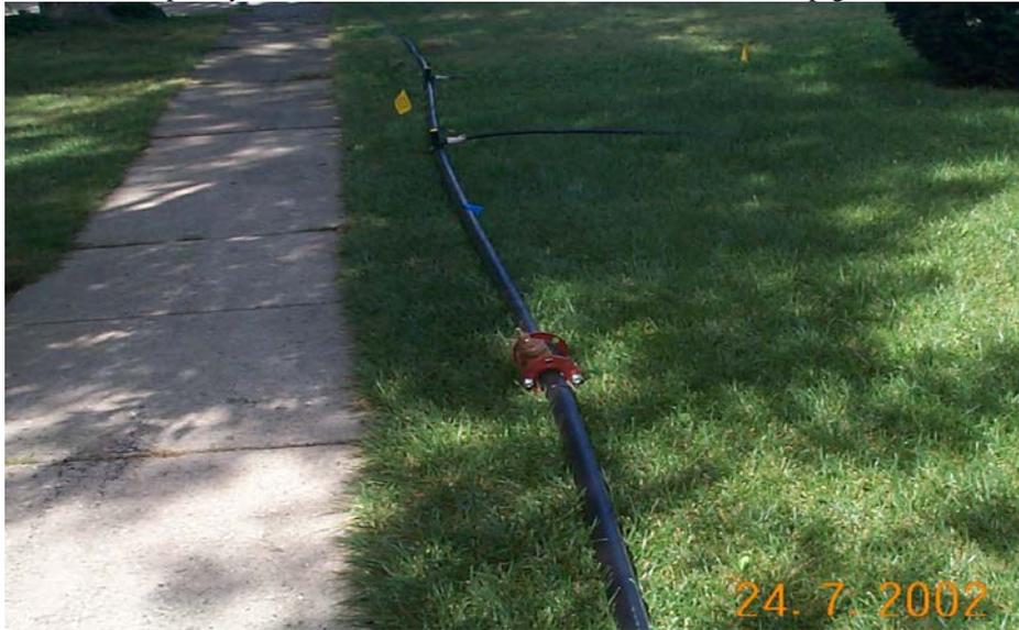
**Figure 20 – 2" HDPE Temporary Water System W/ In-line Valve & Electrofuse Saddles W/ 3/4" HDPE Service Lines**
