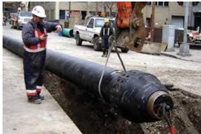
**Figure 17 – HDPE Burst Head**
