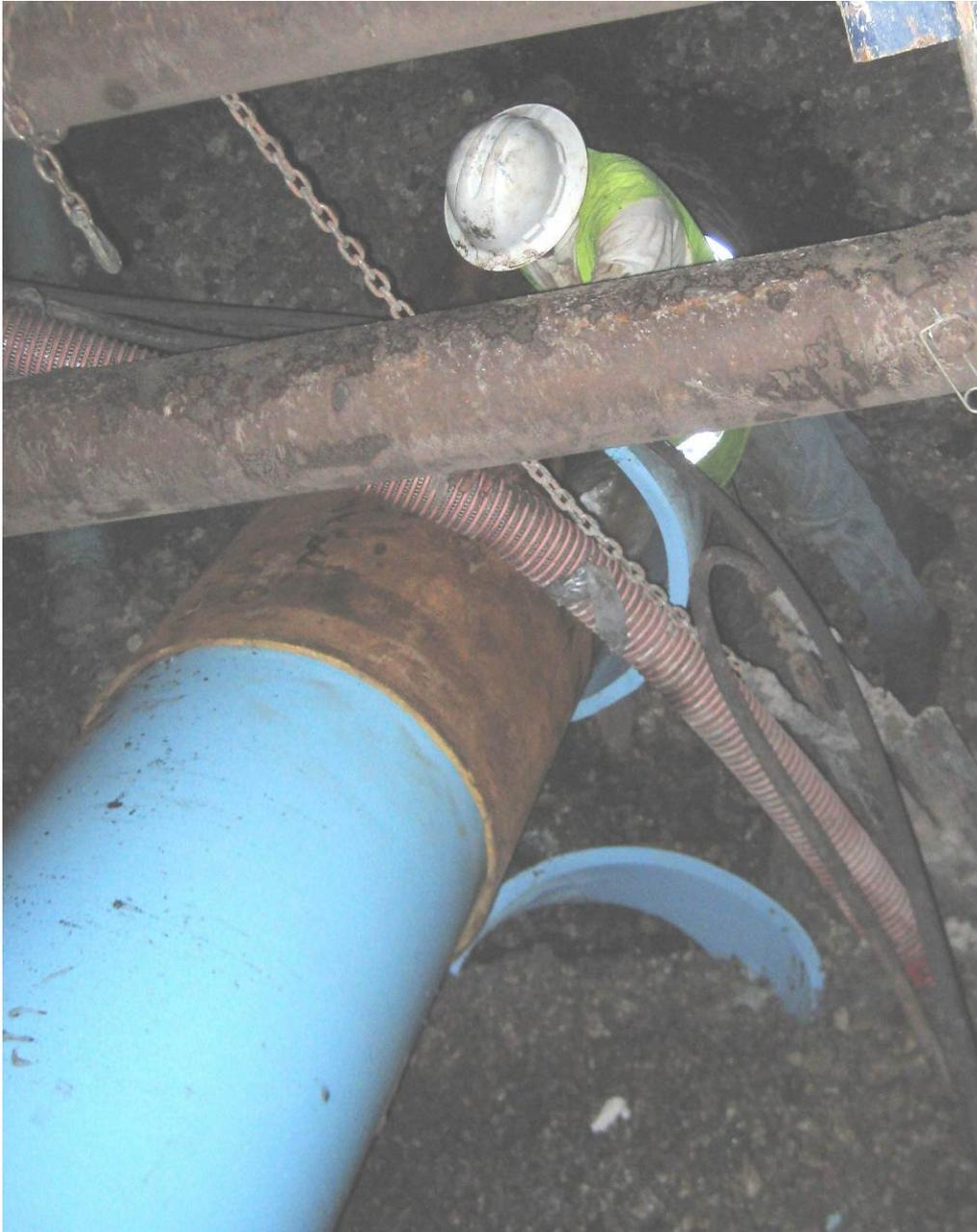
Figure 7. Insertion of the 24-inch carrier pipe into the previously installed 30-inch casing pipe.
