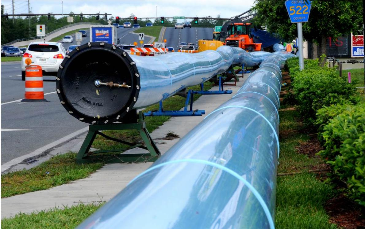
Figure 5. Fusion and staging of the 30-inch FPVCP casing pipe along Osceola Parkway.
