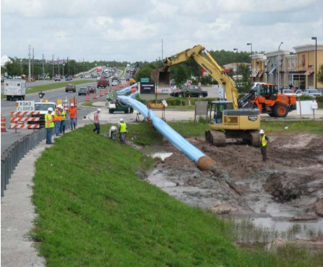
Figure 6. Insertion of the 30-inch casing pipe into the HDD alignment. Note the fusion machine on the left-hand side of the picture showing where the intermediate fusion joints were performed during pull in at Bill Beck Boulevard, which was temporarily closed.
