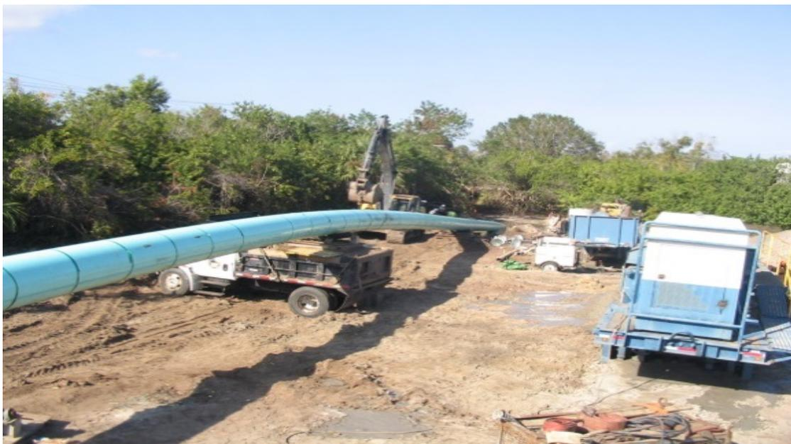
Figure 3: Pipe installation to the south of the wetlands with drill mud recycler setup and telescoping fork lift.
