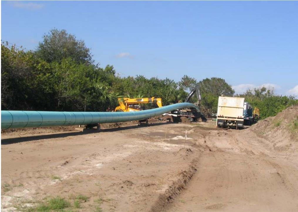
Figure 4: Pipe installation to the south of the wetlands with roller system.
