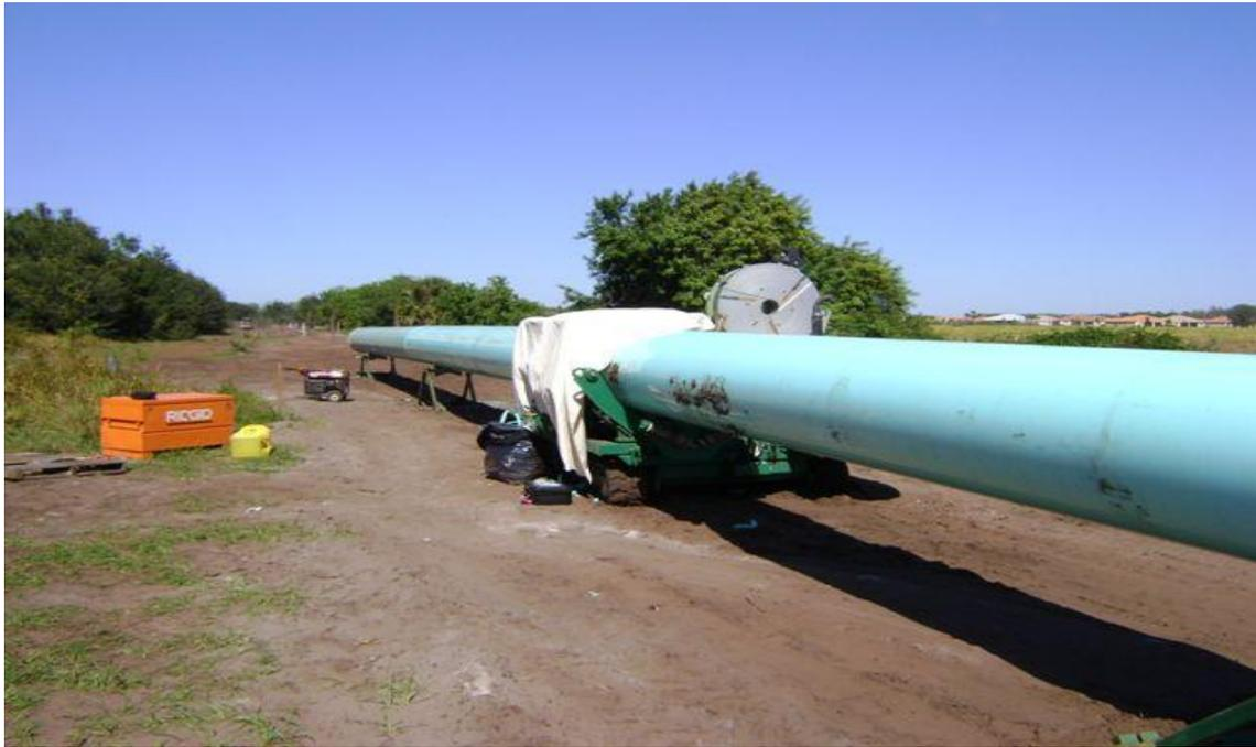
Figure 2: Fusion setup for 2,100 LF of 30" FPVCP force main pipe to the south.
