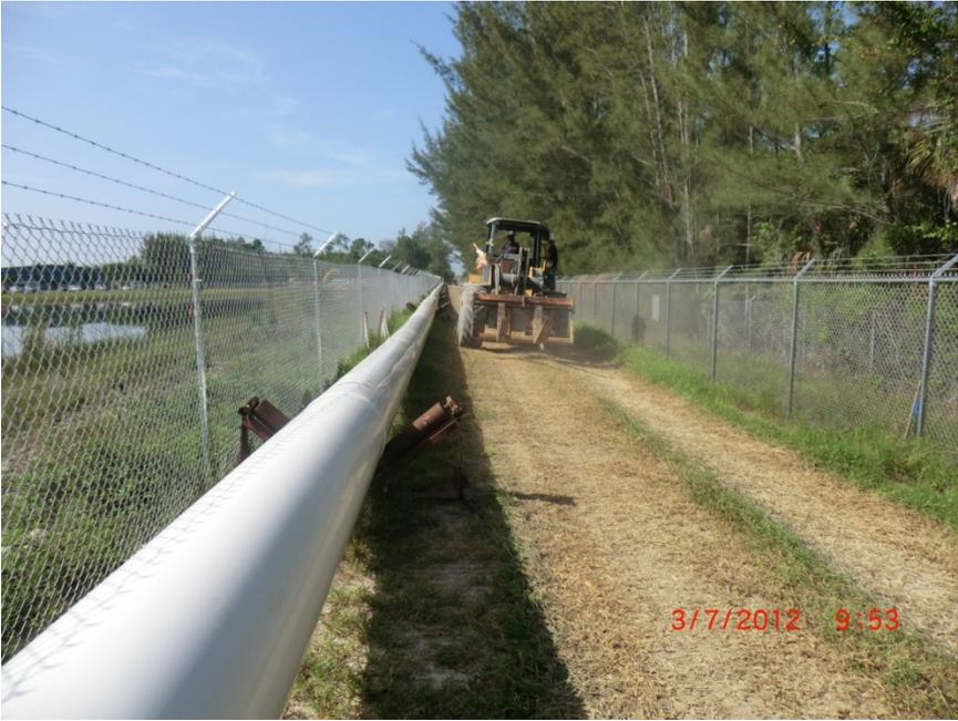
Figure 3. HDD Exit Pit and Staging Area Blocked by Pipe Layout for Long Bore
