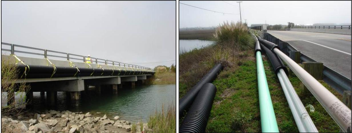
Figure 5. Corrugated conduit sleeves used to support the separate strings of pipe at the bridge location of the laydown area for the crossings. There were three separate sleeves used for each of the utilities, with one housing the multiple AT&T conduits.
