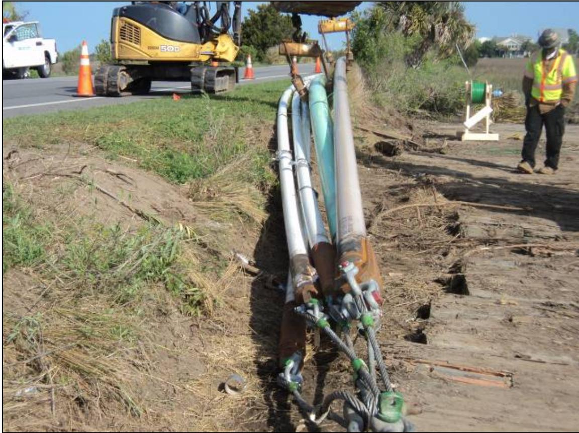
Figure 7. Pipe bundle set up shown as the Folly River crossing is beginning. From left to right are the three AT&T conduits, the sewer force main, and the gas main.
