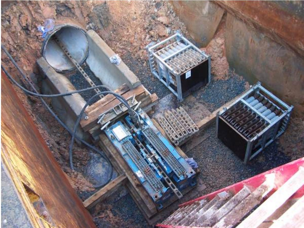
Figure 7. Grundoburst 800G static bursting unit set up and blocked in place in the receiving pit to pull in the new pipe. The steel rods are shown in the machine as well as in their storage packs for removal from the pit.
