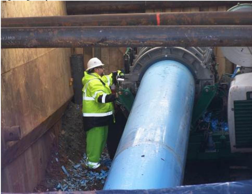
Figure 5. Length of FPVCP being thermally butt-fused within the pit.
