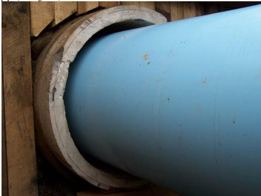
Figure 6. Close up view of new FPVCP inserted into the existing PCCP.
