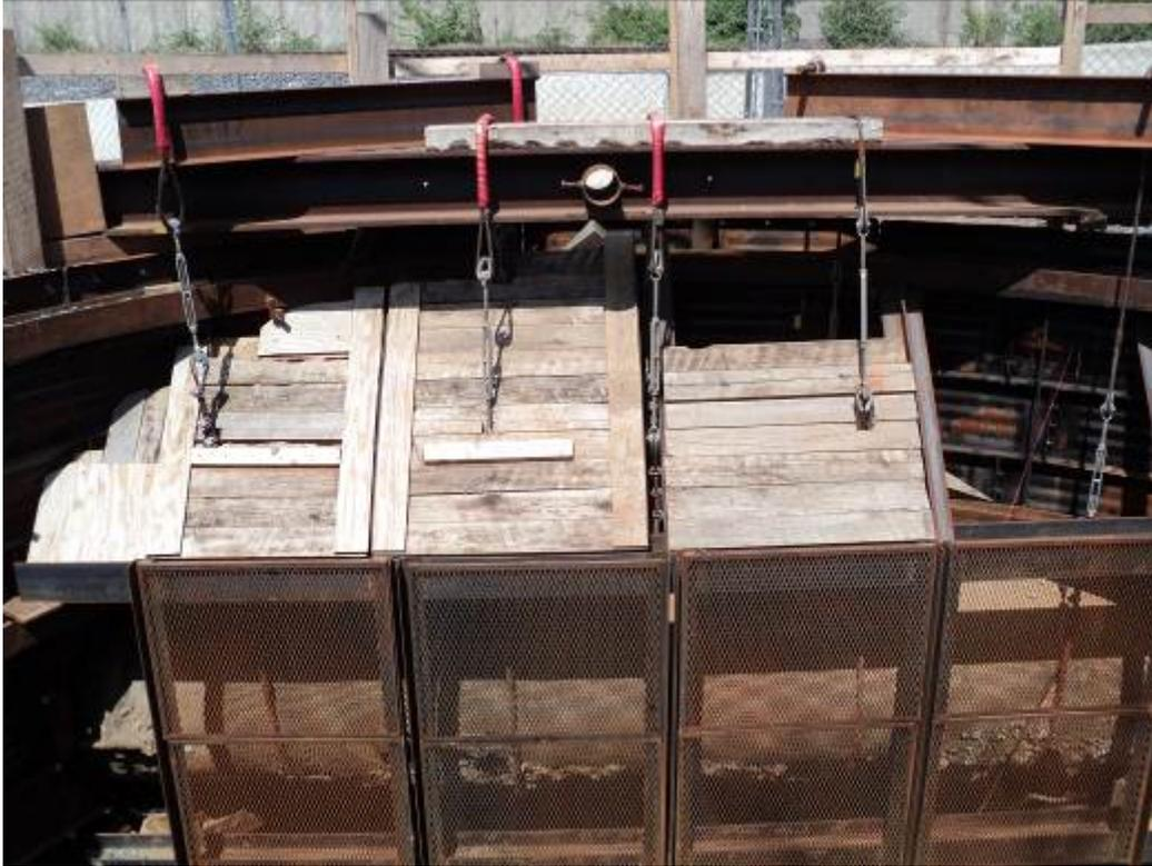
Figure 8. Protection of the 36-inch PCCP within the shoring system.
