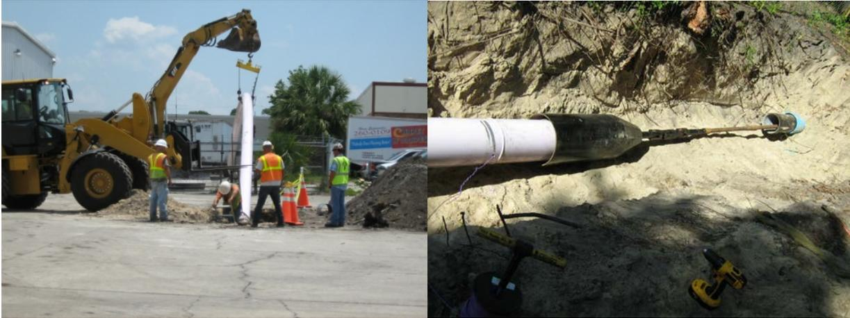
Figure 2. The picture on the left shows an elevated alignment of the replacement pipe being installed with pipe bursting methodology, and the picture on the right is a close up of the pipe bursting head, expansion head and replacement pipe as it is entering the existing pipeline.
