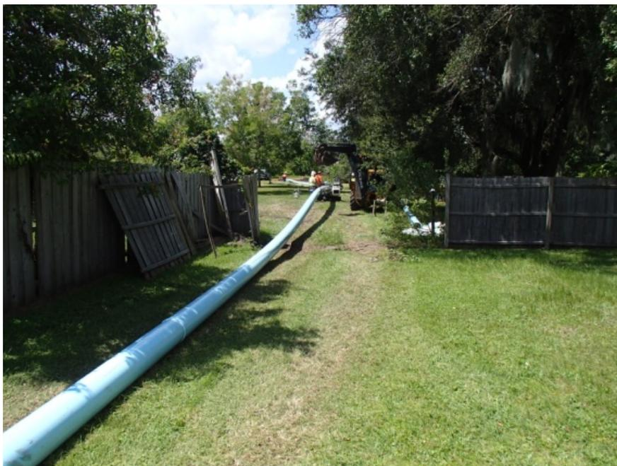
Figure 5. The pipe for the HDD was fused and staged in a tight landing area on one side of the spillway.
