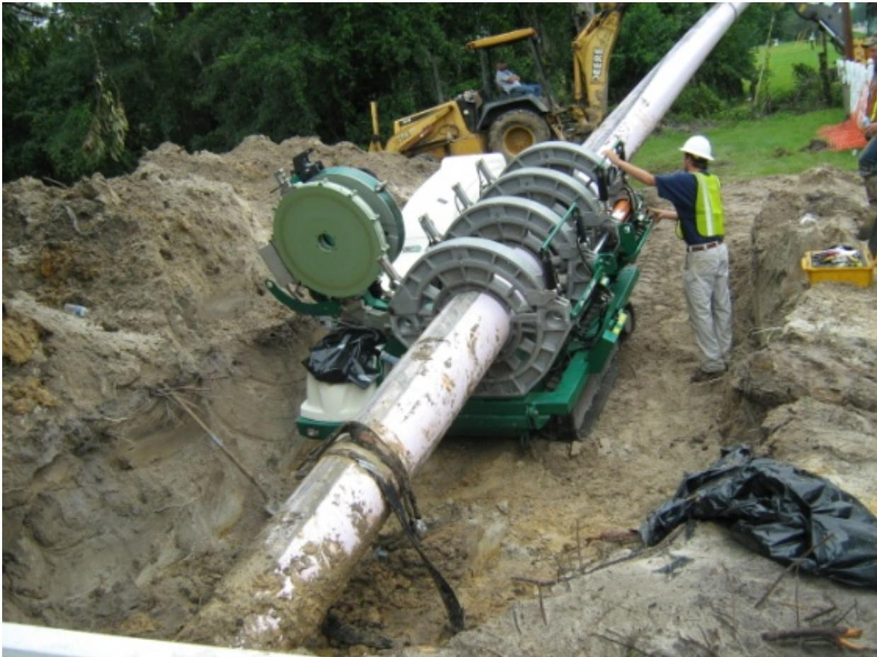
Figure 3. An intermediate butt-fusion joint is performed at the location of a break that was realized during installation of the pipe string.
