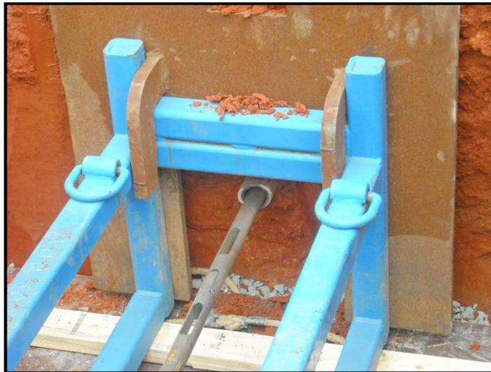
Inserting 1.4-inch rods into existing 2-inch cast iron pipe
