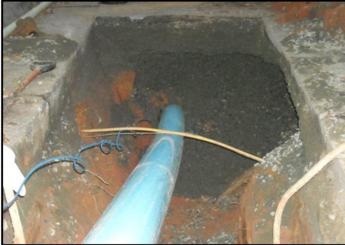
Insertion of replacement pipe with tracer wire
