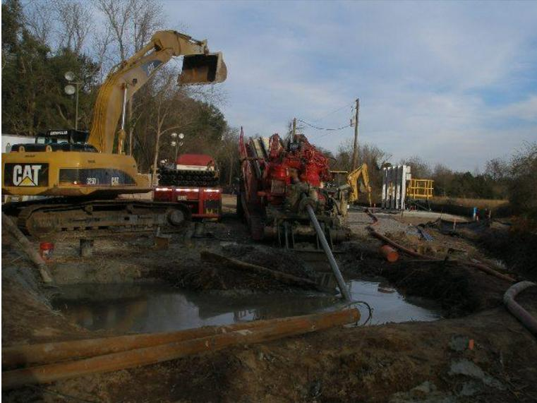
Figure 8. Drill rig and operations of rig side of Stono River crossing.
