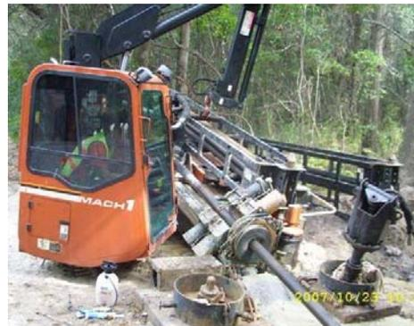
Figure 11. BoreTek's Drill Rig being utilized for the 24" DR 25 Fusible C-905 installation by HDD.
