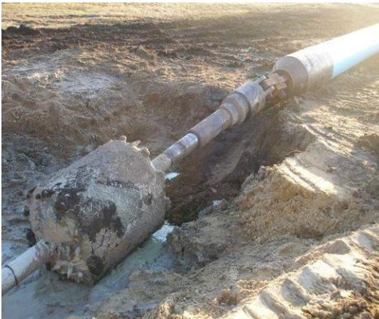
Figure 5. Pullback reamer and pipe pull-in assembly
