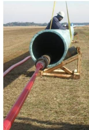
Figure 7. Ballasting operation
