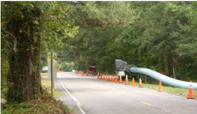
Figure 10. Fusion Machine and Fusion Layout. Large tree on left is an example of the project site protected by the trenchless work.
