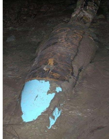
Figure 9. Pullhead and pipe recovery after successful installation.
