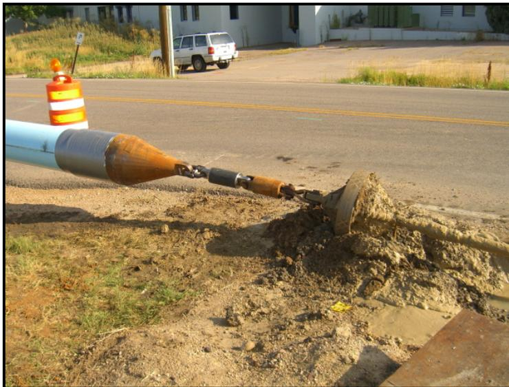
Figure 9. TensiTrak™ In-line Pull Force Measuring Device
