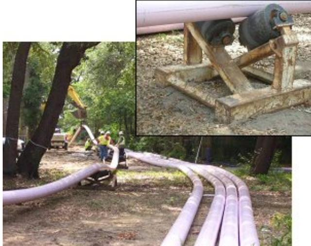
Figure 2. Fusible PVC™ Pipe on Rollers
