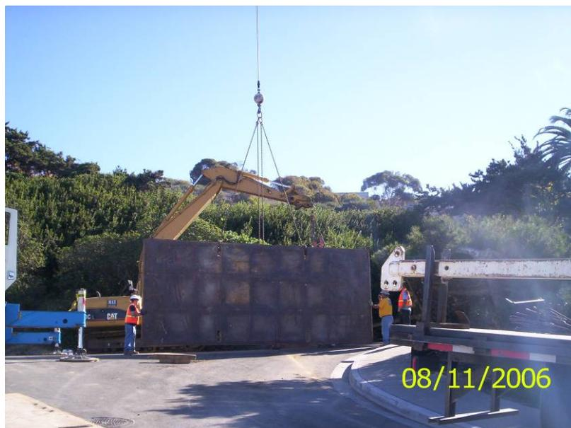
Figure 3 – Installing Trench Shoring at a Pit Location
