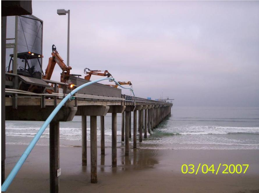
Figure 5 – Installing the Pipe from the SIO Pier
