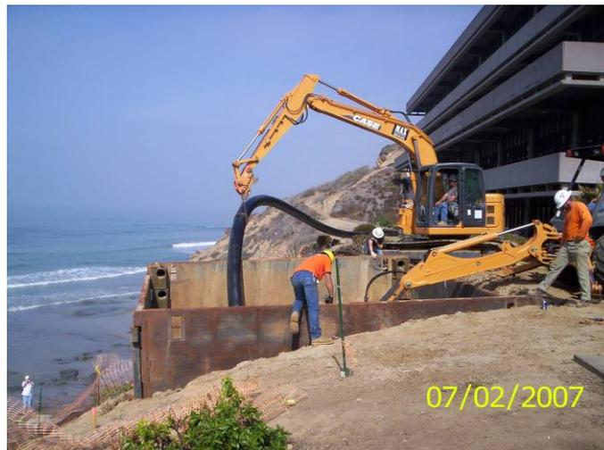
Figure 6 – Installing welded pipe on top of a high embankment
