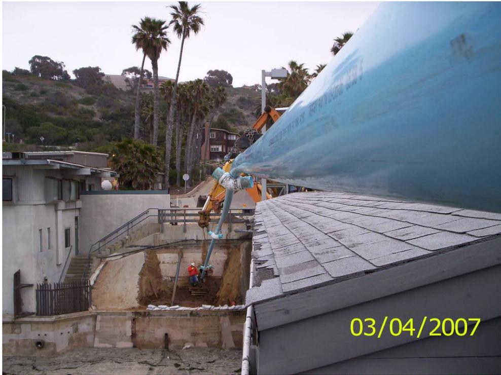
Figure 7 - Pulling the Fusible PVC™ Pipe String Through the Seawall
