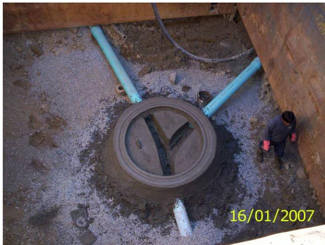
Figure 8 – Base of a Seawater Discharge Manhole
