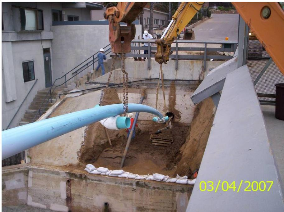
Figure 6 - Pulling the Fusible PVC™ Pipe String Through the Seawall
