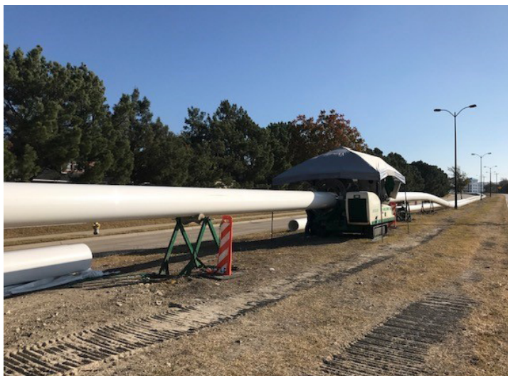
Thermal butt-fusion assembly of Fusible PVC® pipe
