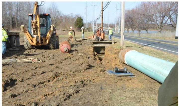
Preparing the insertion pit for the Fusible PVC® pipe at the end of the borehole
