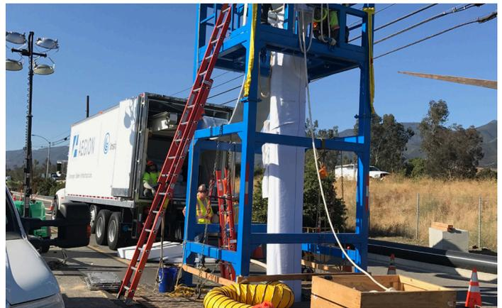
Engineered steel frame set at grade and secured in place for installation of the CIPP
