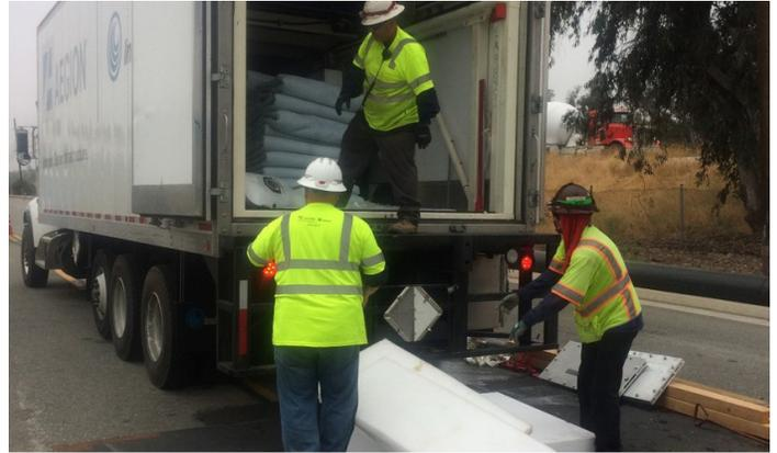
Pre-inverted CIPP downtube secured to the top of the conveyor and locked into position inside of the refrigerated transport, ready for installation
