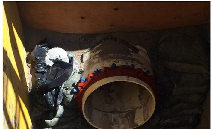
Deflected 24-inch PVC brine line was temporarily rounded using a megalug fitting. Installation of the InsituMain® CIPP permanently rounded and stabilized the PVC pipe.
