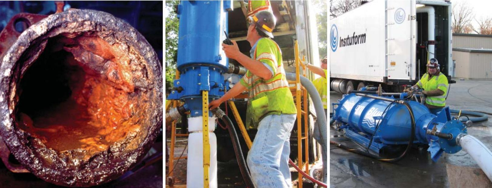
**The InsituMain<sup>®</sup> system is ideal for the renewal of force mains and other pressure pipelines up to 96-inches in diameter.**
