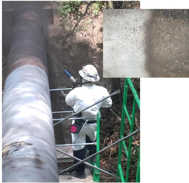
**Figure 6: Surface Preparation of Host Pipe**
