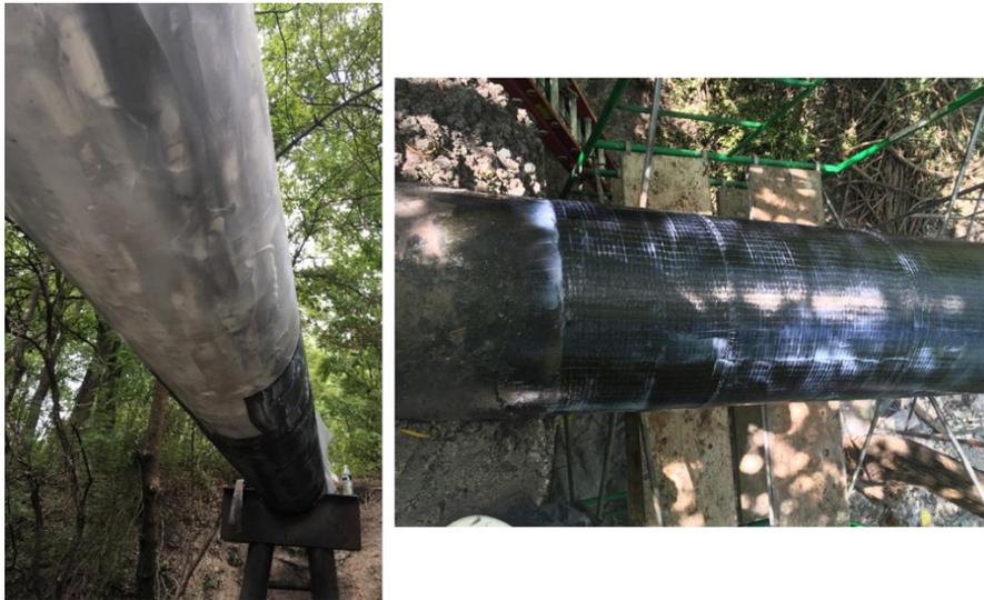
**Figure 7: Installation of CFRP System**
