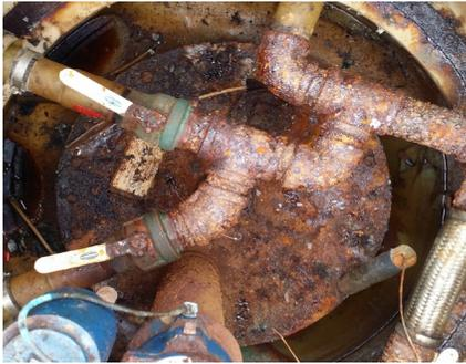
Sump corrosion caused by Ethanol and Acidic Vapor.
