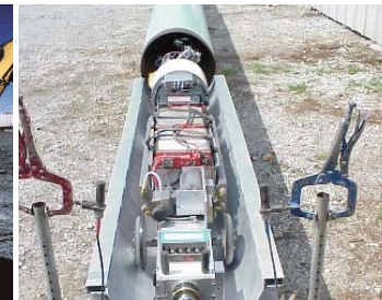
Robotic Interior Weld Coating
